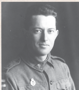
Photo courtesy of Michael Stephens
